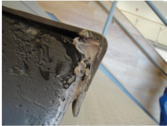
Stair tread that is laid as shown in the picture above will break at the nosing due to repetitive flexing.
